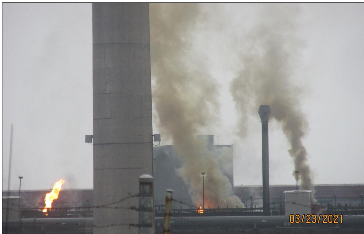
Photo 17: Flaring and release of raw coking gas from 8 Battery standpipes and pushing operations releasing raw coke gas (far right)
