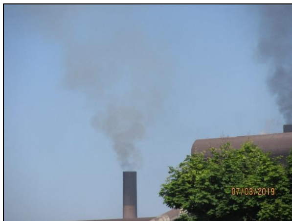
High opacity 8 Battery COB stack
