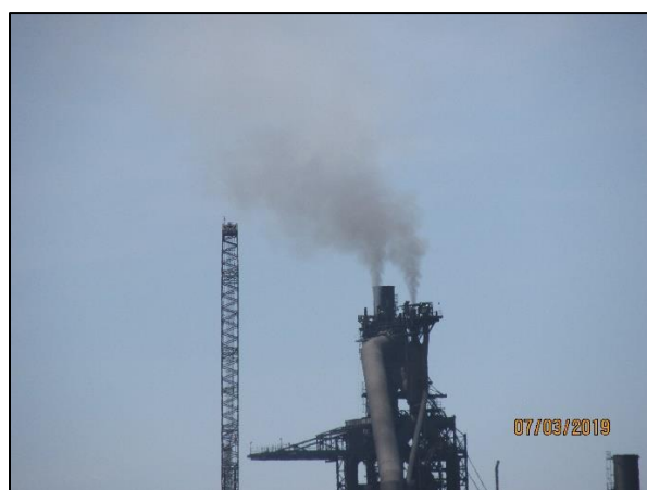
No. 7 Blast furnace dirty bleeder valve emissions
