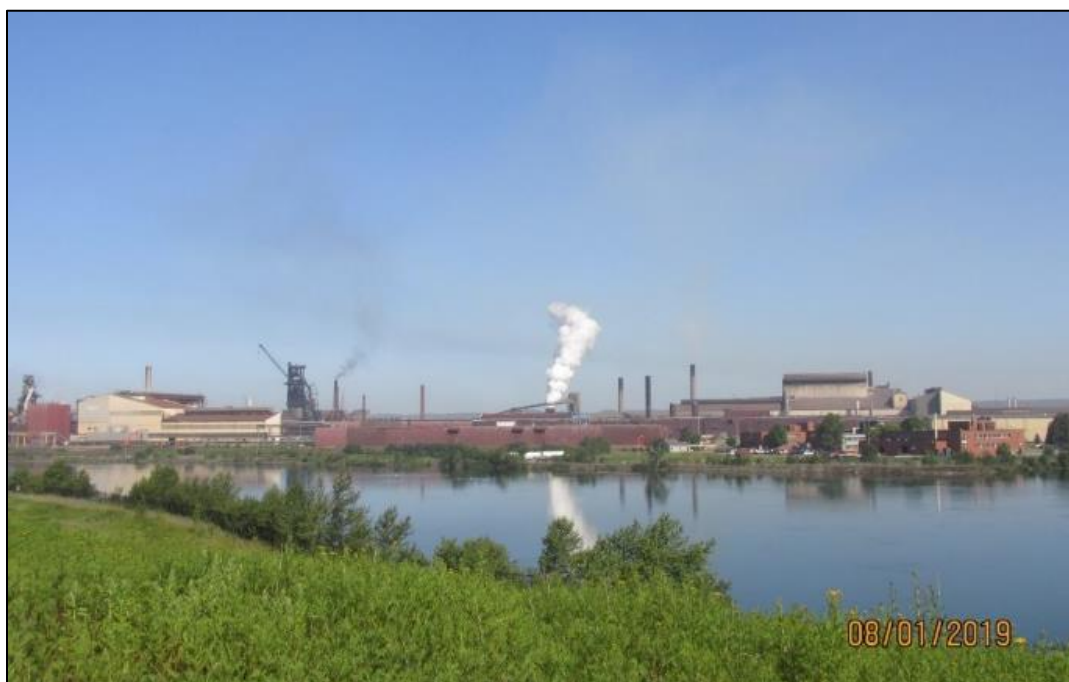
Photo 30: High particulate haze. Quench Tower still operating seen by the white plume @11:24 am
