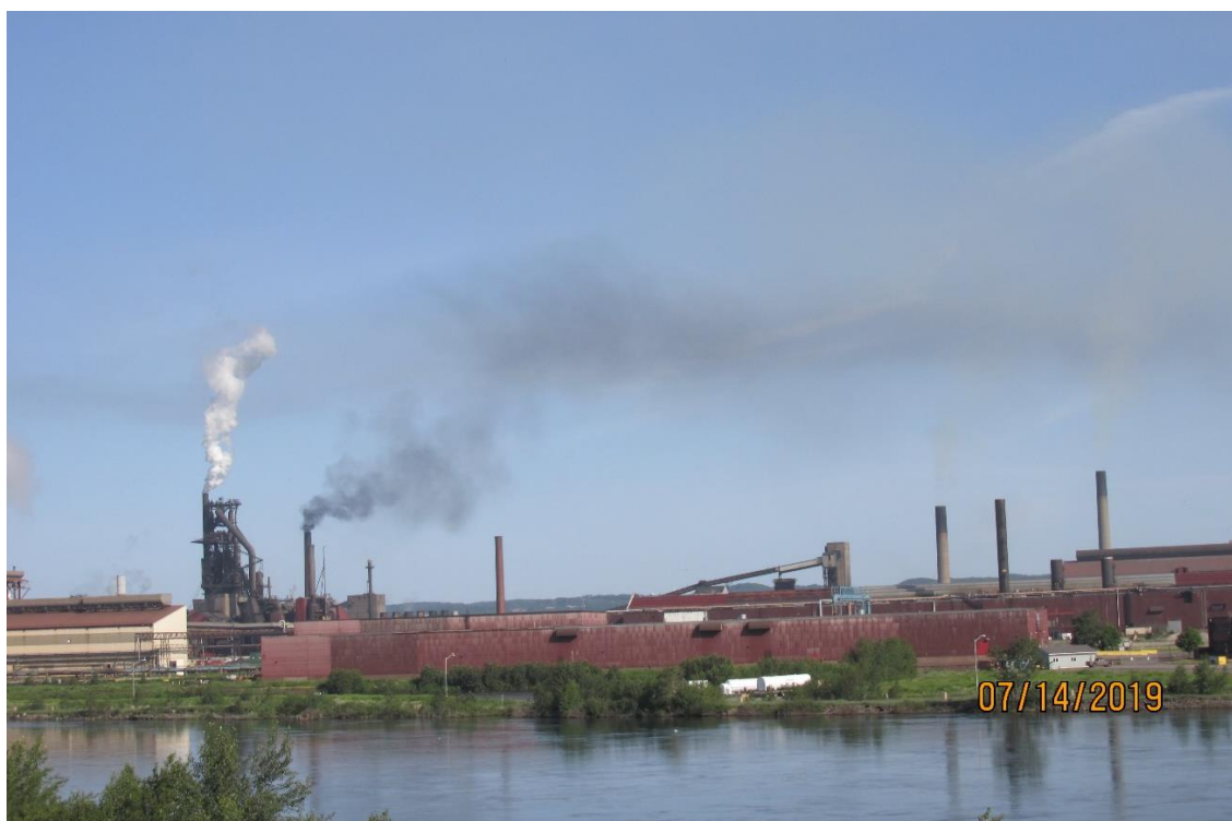
Photo 24: Dark stack emissions from 7 battery and pale yellow from 8 and 9 COB stacks @ 9:11 am
