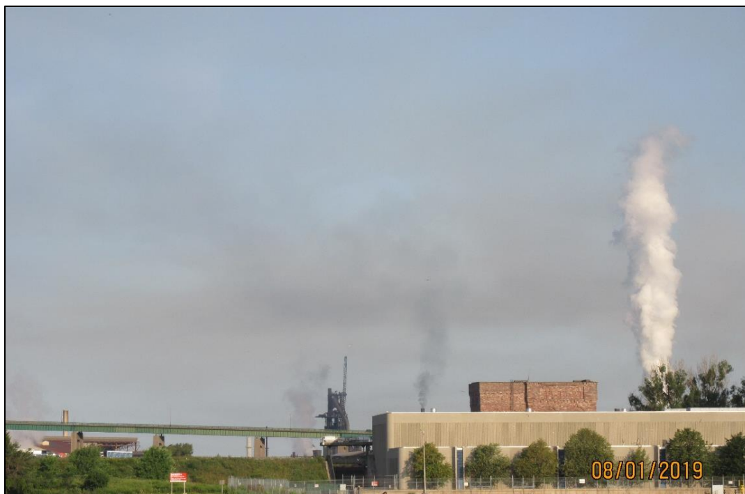
Photo 29: High particulate haze. Quench Tower ("Quencher") was operating seen by the white plume (far right) from pushing operations @ 7:54 am.
