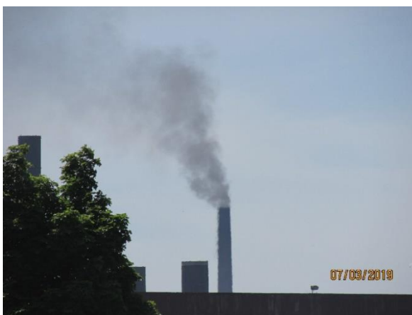
High opacity 7 Battery COB stack
