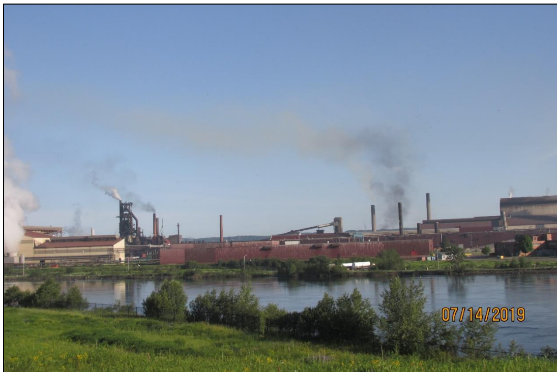
Photo 21: Pale yellow stack emissions and pushing emissions from 8 Battery @ 7:59am
