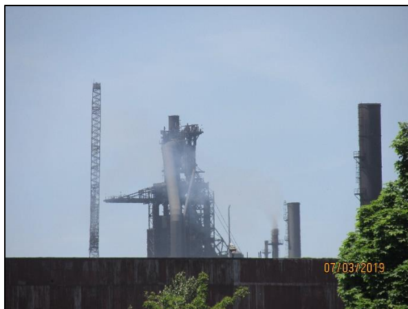
Particulate released from NO.7 BF flare stack
