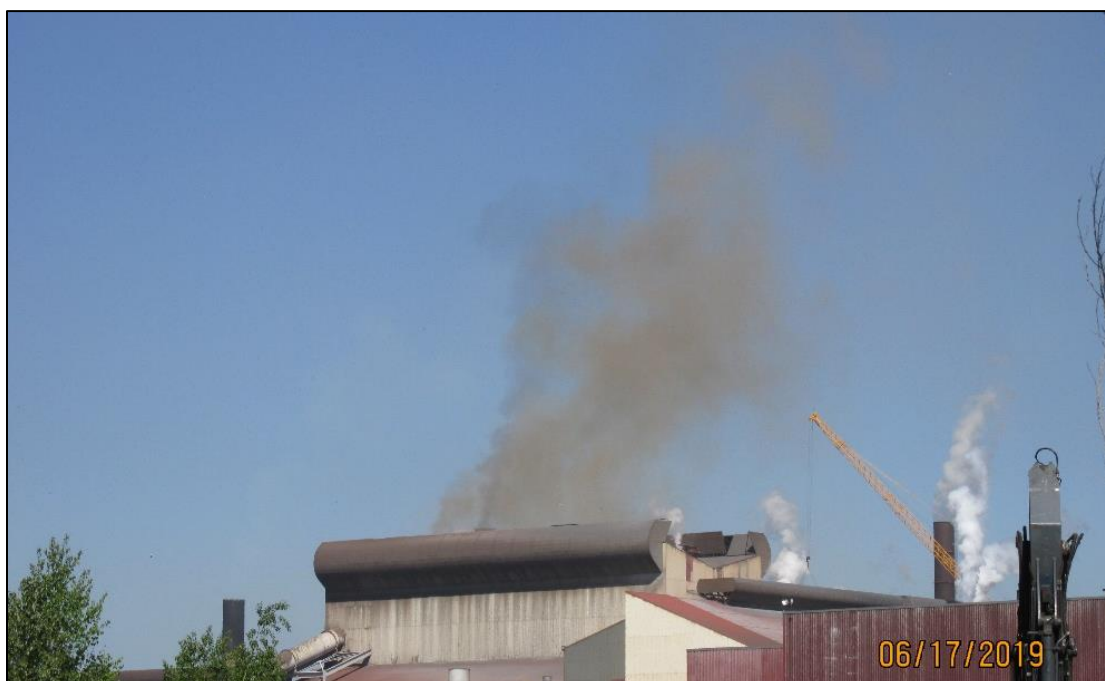
Photo 10: Multiple fugitive iron emissions from the rooftop of the No. 2 BOSP
