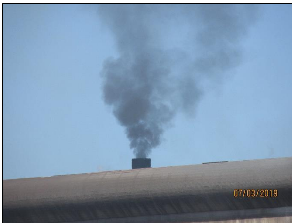
High opacity 9 Battery COB stack
