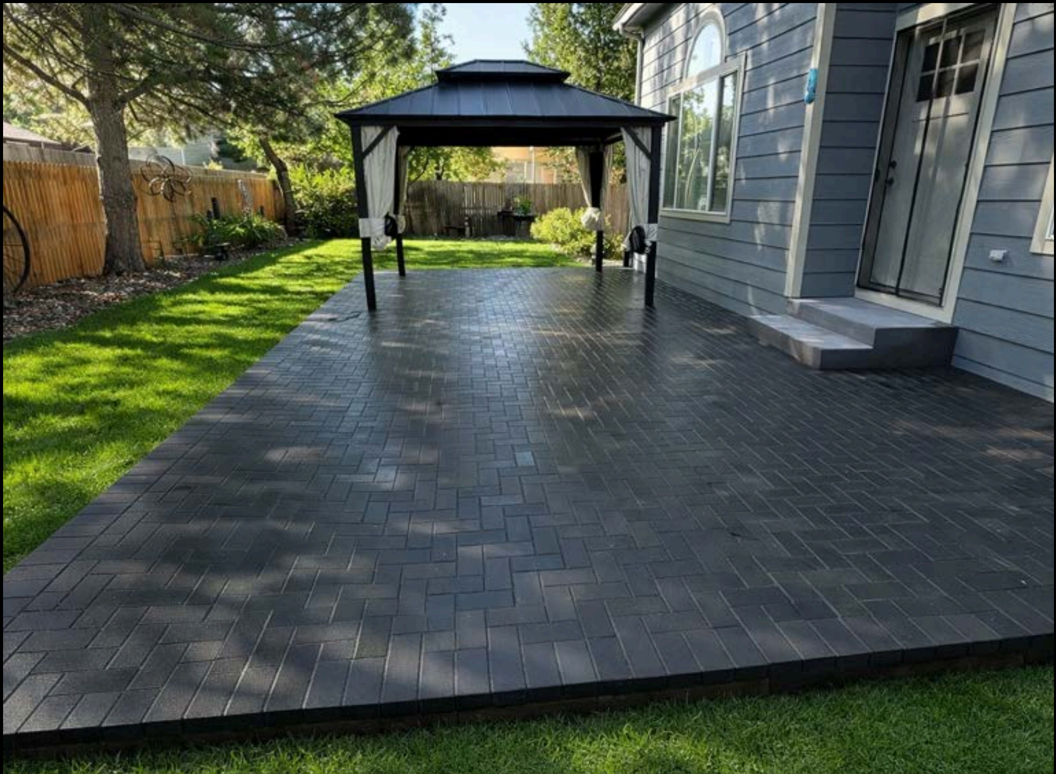
MODERN PAVER PATIO | CONCRETE STEPS | OUTDOOR PAVILION INTEGRATION
