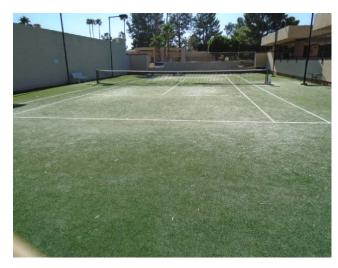
General Acrylics installed a Nova ProCourt XP sand-filled tennis court surfacing system over the asphalt tennis court in early 2016 for \$32,480. We have been advised to budget to replace this type of court system on a 20 year cycle.
