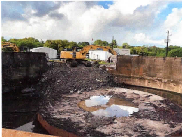
Demolition of Original WWTP
