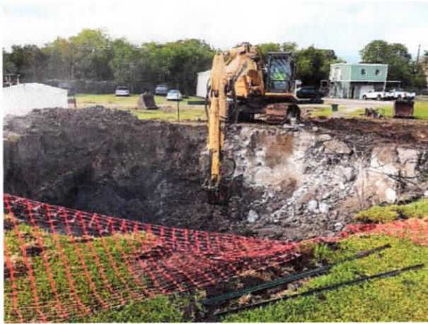
Demolition of Standby Clarifier
