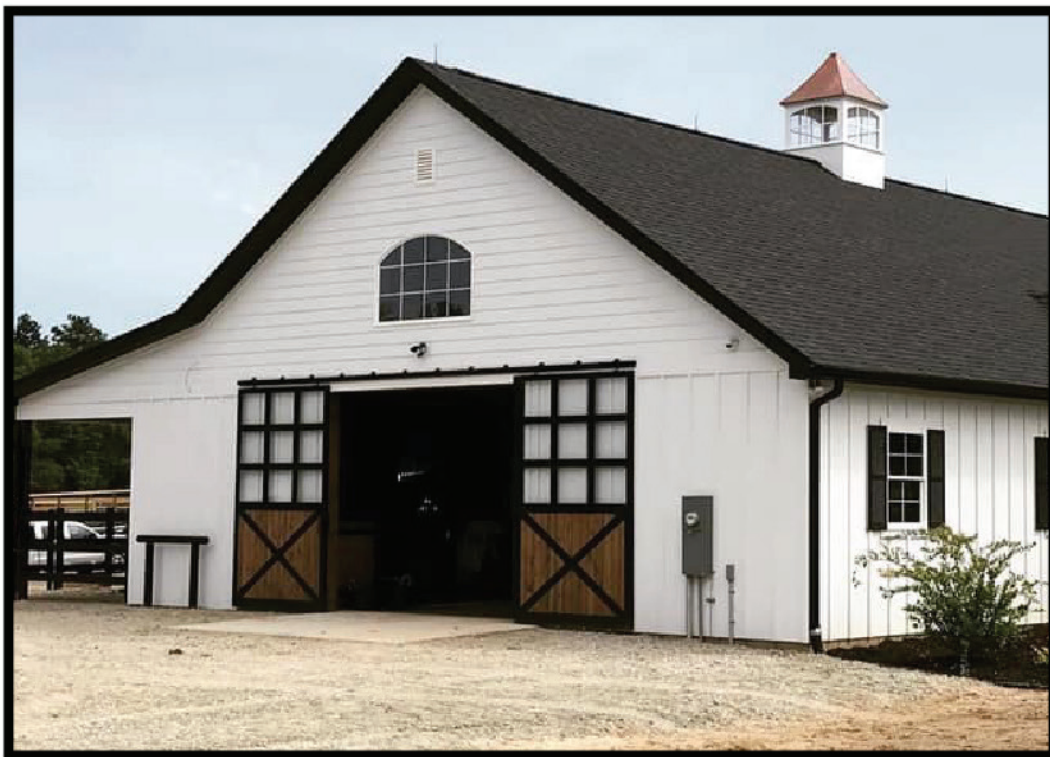
9 Light Glass Topped Barn End Door with Vertical Wood Fill & Cross Bucks
