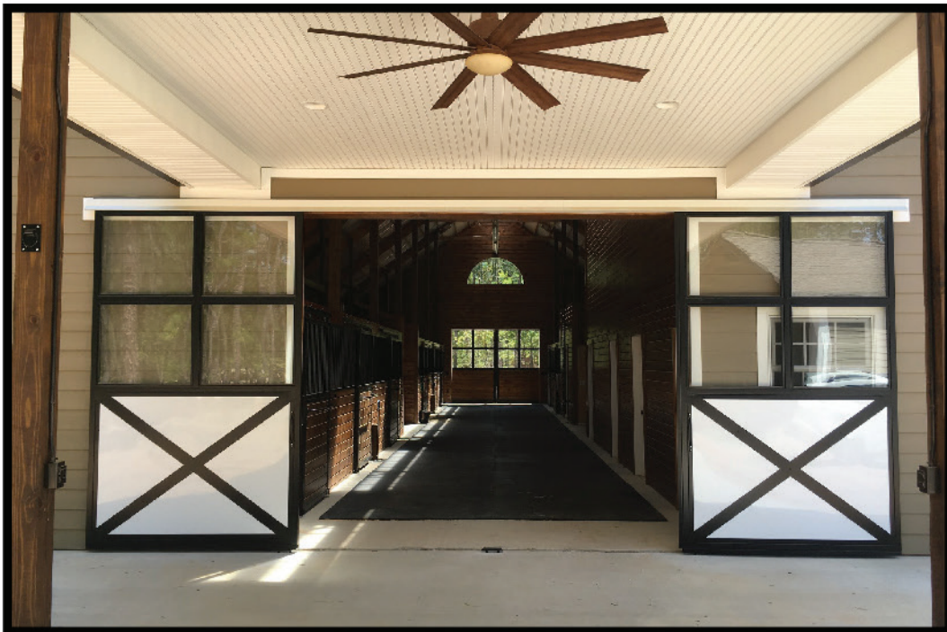
Quad Glass Topped Barn End Door with Bottom Cross Bucks & Powder Coated Filler Panels
