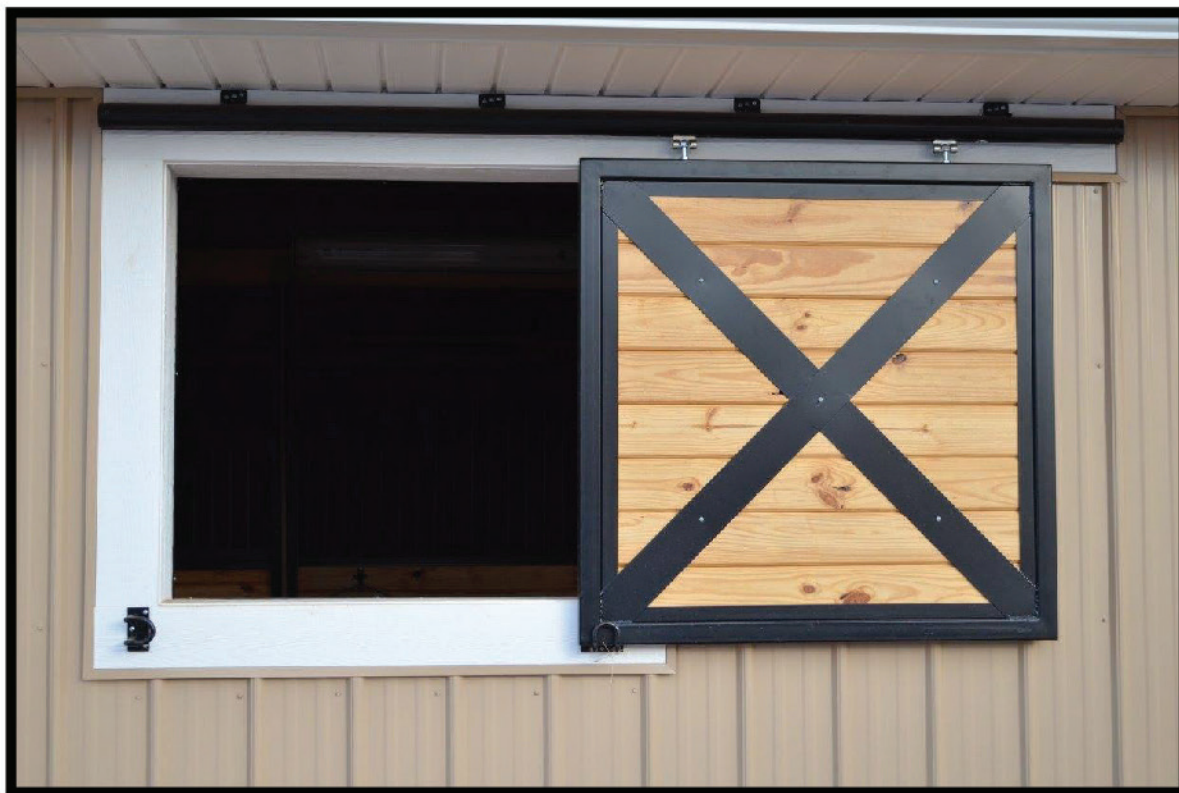
Sliding Window with Horizontal Wood Fill & Cross Buck
