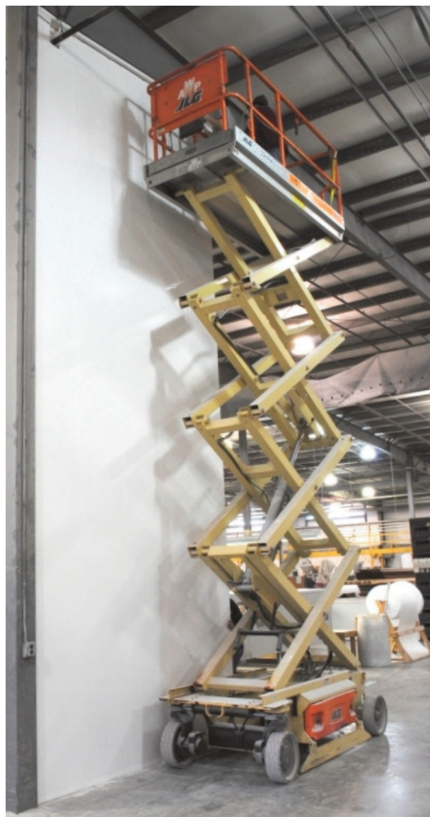
24 Foot High Partition Wall Installation
