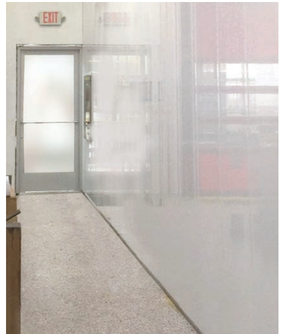
2-1/4" P224 Partition Wall Installation
