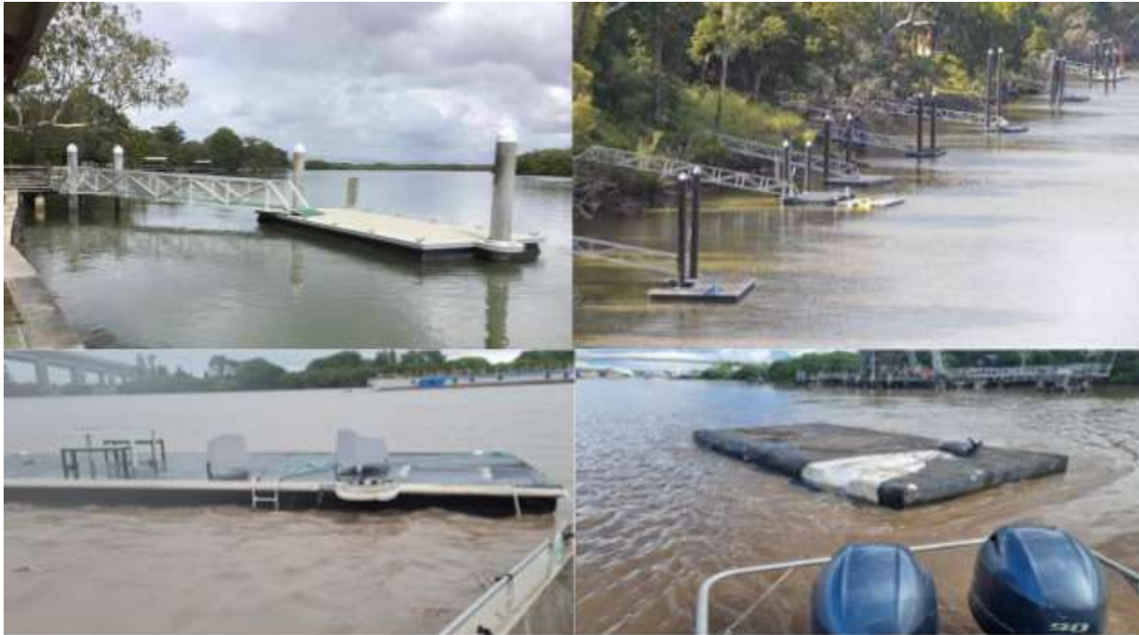
Figure 8. Images of pontoons in the Brisbane River before the 2022 floods (top) and during the flood (bottom), Image credit: Ocean Crusaders.
