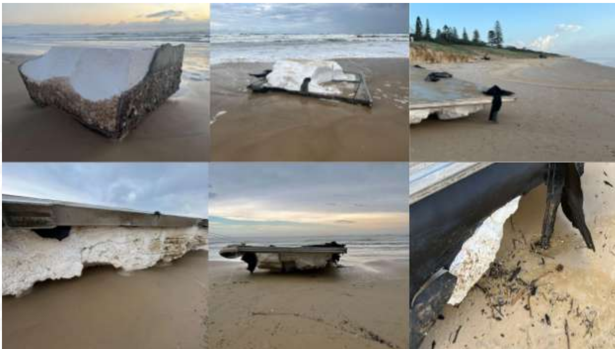
Figure 9. Examples of breached or absent encasement of polystyrene pontoons that were beached following the 2022 floods. Image credit: Sharyn Kerrigan
