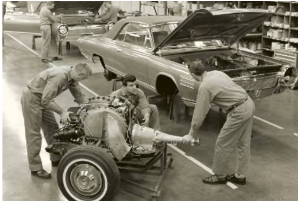
1963 Turbine engine installation
