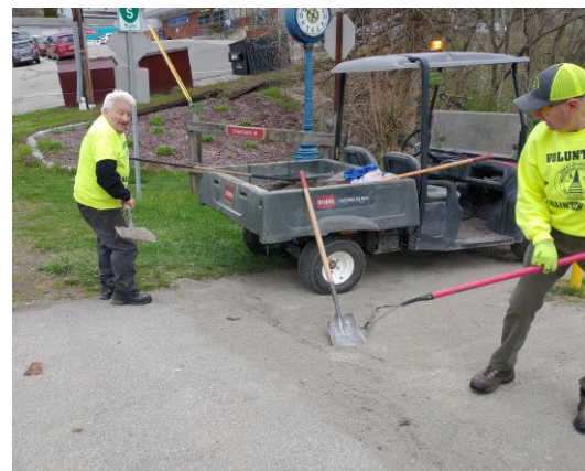
John Brunory & Rick Hornick repairing the trail in West Newton
