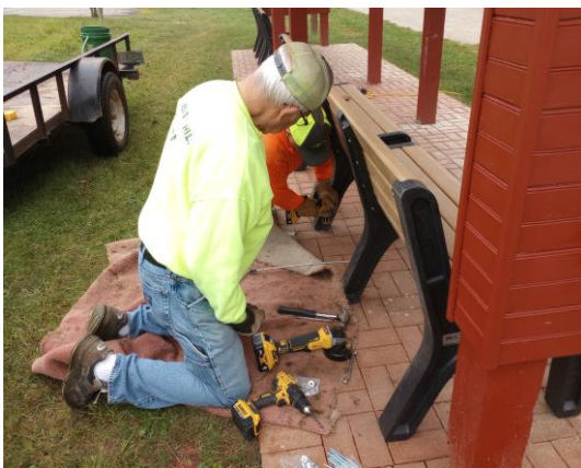
Jim Lockschmidt & Marty Fao installing Benches in Memorial Pavilion
