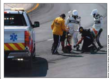
Workers patch an area of track pavement at New Hampshire Motor Speedway during a break in the action Sunday.
