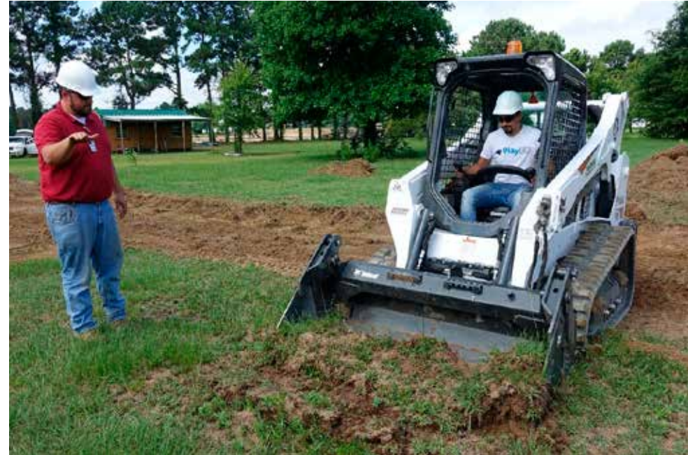
Grady instructs students on how to strip the vegetative layer before digging footings for a house
