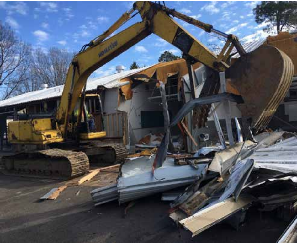
Workers make way for SCC's new welding facility
