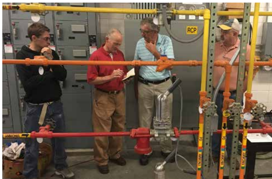
SCC Ammonia refrigeration instructor Leerkes (third from left) shows off the facility to Sanderson Corporate Maintenance Managers, Norman Butts (second from left) and Dean Jackson (R). Current student, Tevlen Murphy from Smithfield company's Tarheel Plant, observes.
