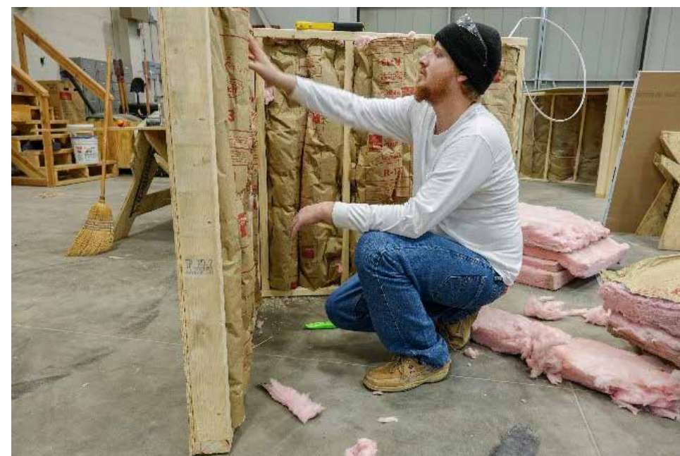
A student installs insulation in the Construction Systems Technology program at SCC. There is a great deal of correlation between current SCC programs and upcoming programs. (Cheyenne McNeill)
