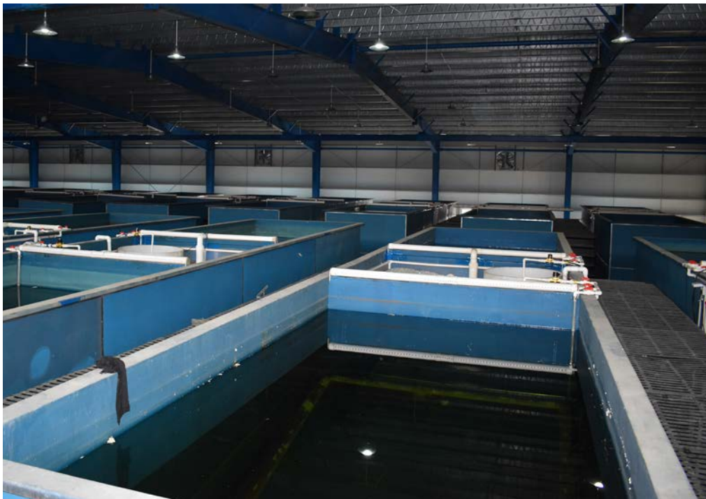
Recirculating aquaculture facility under construction in Guangdong province, China.
