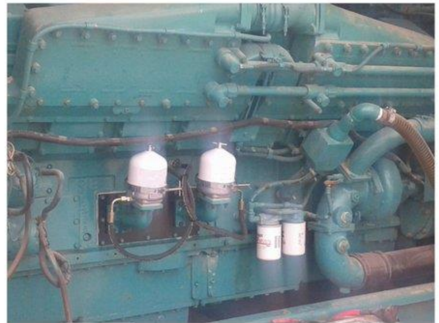
Cummins KTA50G Genset with Dieselcraft OC-50 Direct Mount Oil Centrifuges
