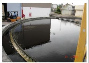
A waste-water treatment had sludge bulking problem in final clarifier. After trouble-shooting and optimization, the plant ultimately complies with standard B effluent discharge standard.
