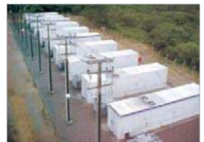
Fig 8.4 - Cummings Generators in Manaus
