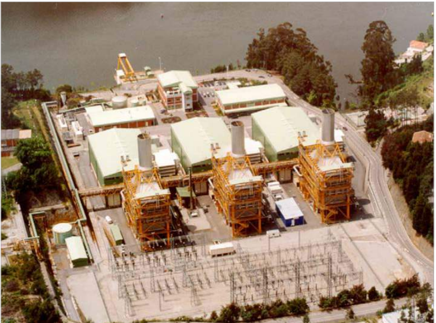
Figure 1.8 - Tapada do Outeiro (Combined Cycle Gas Turbine Power Plant)
