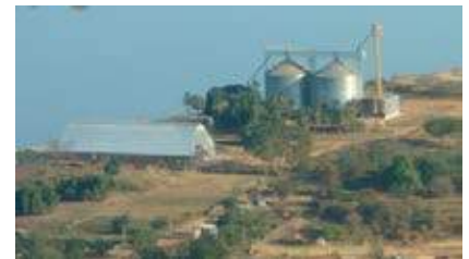
Figure 6.2 - Ibotirama Harbour Unit
