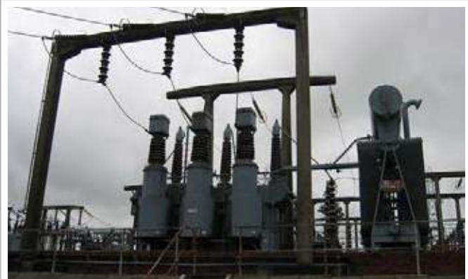
Figure 7.14 - Example of a thermal-powerstation step-up substation
