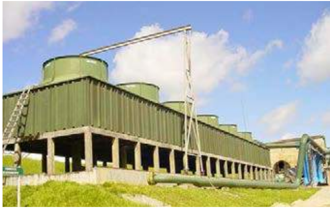
Figure 7.10 - Wet-type countercurrent cooling towers
