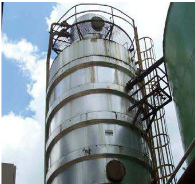
Figure 7.11 - Vertical atmospheric-type deaerator
