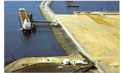
Fig 8.1 - Continuous Self Unloader Ship at Sines Port
