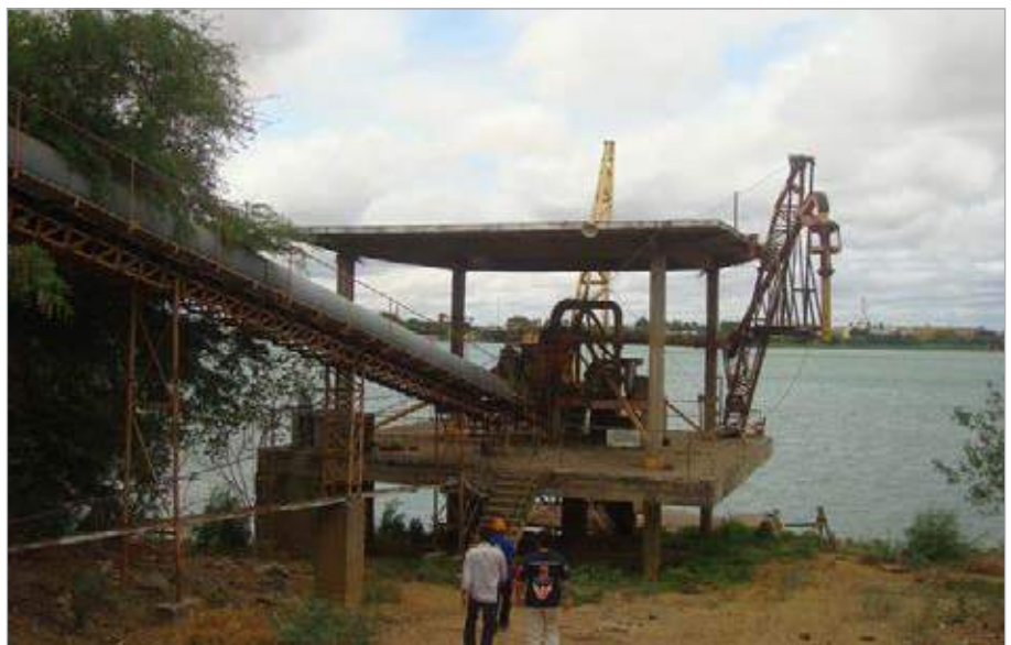
Figure 6.5 – Loading Dock at Petrolina Industrial Unit
