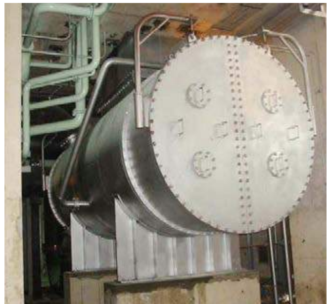
Figure 7.9 - Shell and tube-type condenser
