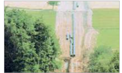
Fig 1.4 - Primary Gas Pipeline Project (Portugal)
