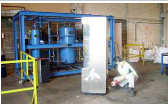
Figure 9.4 - 1st Phase Gas Reclamation Plant
