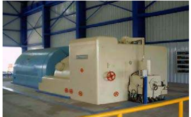
Figure 7.8 - Condensation turbine: turbine in foreground, coupled generator in background
