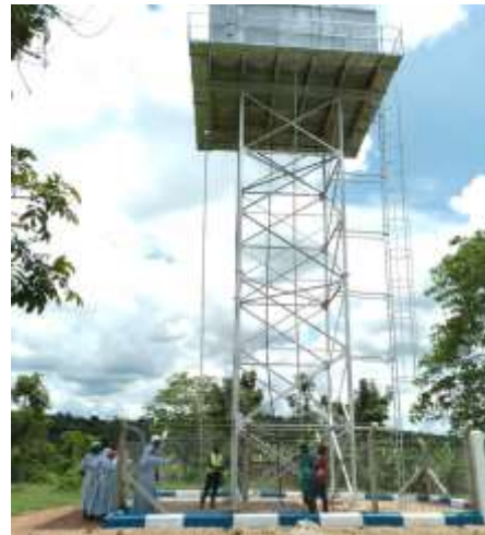
Inspection of the water supply tank & fence
