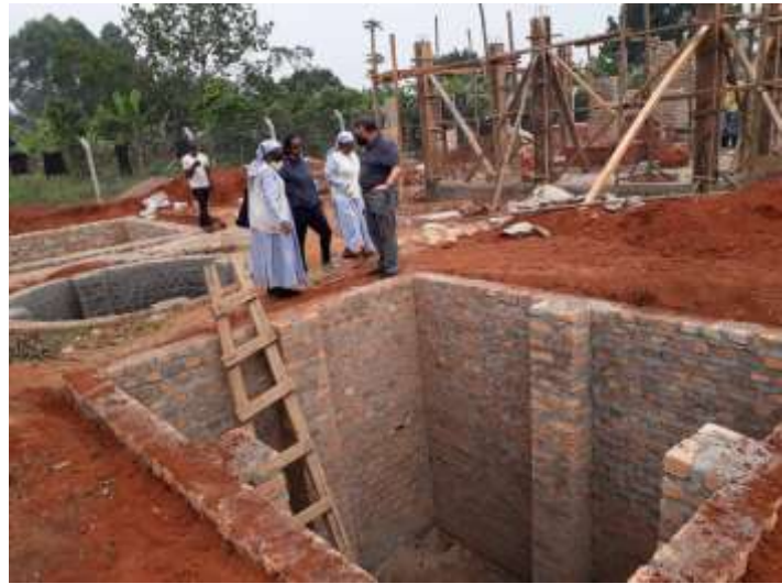
Beth & Michael's visit at the Medical Waste Management project
