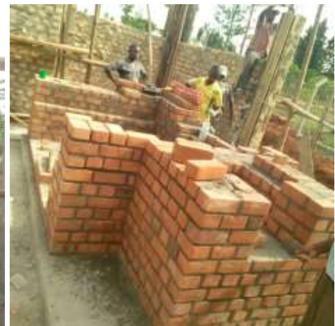
Construction of the incinerator
