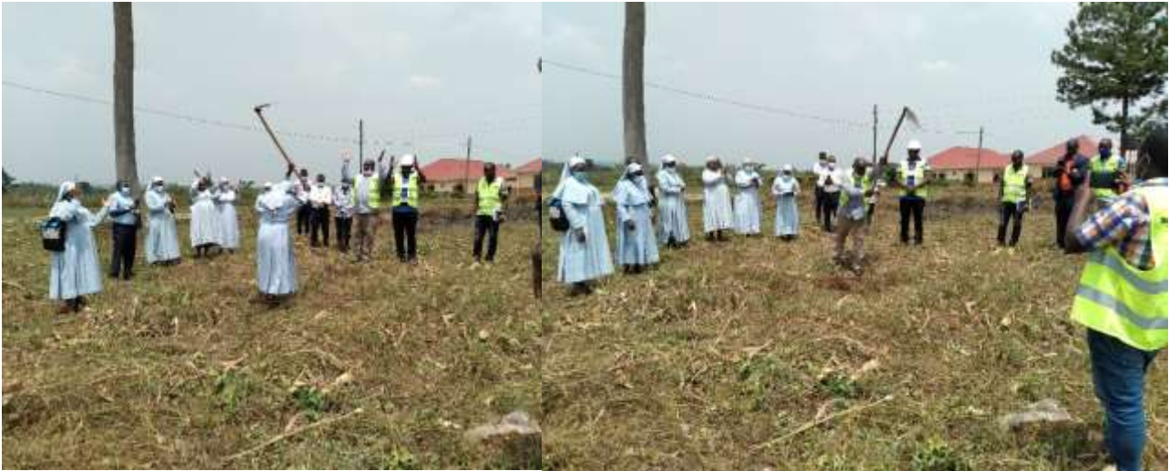
The Mother General and the Contractor breaking the ground
