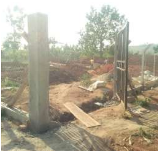
Chain-link Fence with Gate
