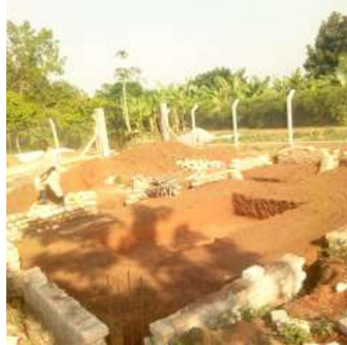
Foundation of the incinerator
