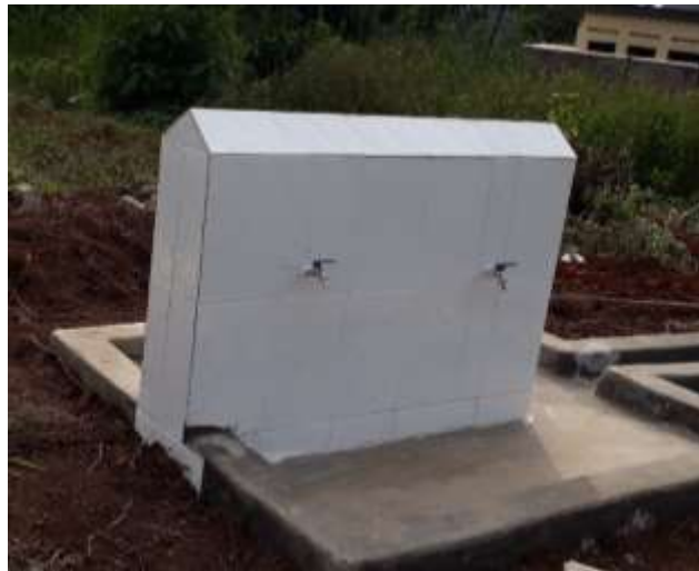
Completed Water collection points
