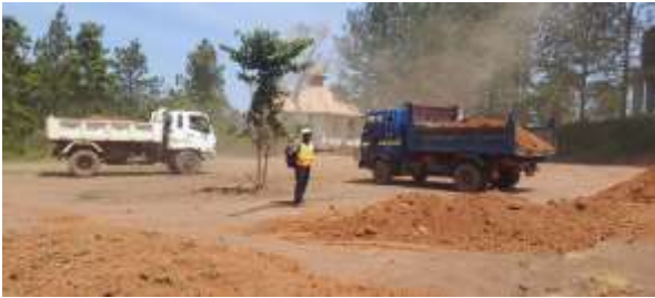
Dumping marram in the parking yard
