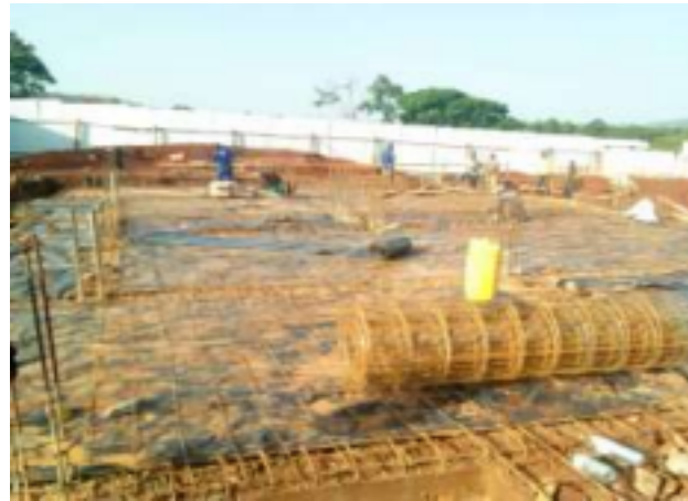
Guest house – backfilling works Doctors' House - Installation of BRC and DPM
