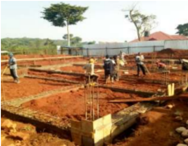
Guest house – backfilling works Doctors' House - Installation of BRC and DPM
