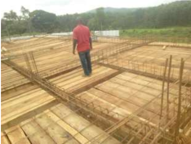
Steel works on Doctors' House
