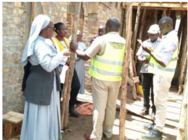
Art Janet inspects construction projects at Rwibaale H/C
