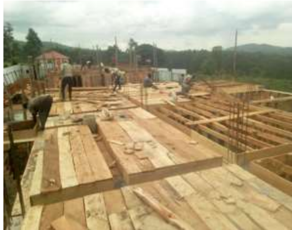
Slab Form Work on Guest House
