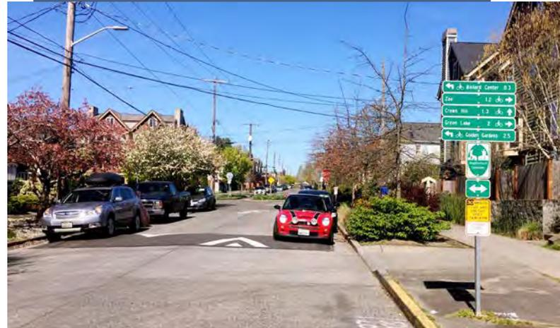
Speed tables are a proven traffic calming treatment that are preferred for emergency vehicle access over speed humps. They should be placed at 350' intervals. This treatment is designed to achieve vehicle speeds of 18-20mph, and are different from speed bumps commonly used in parking lots.
