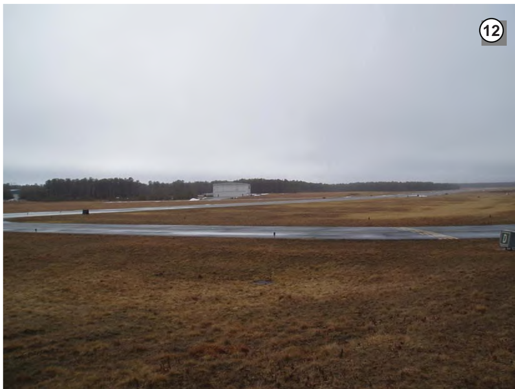
Looking southwest from the east side of the Airport toward Building 18 in the distance (Field Photograph P1010014, February 27, 2013).
