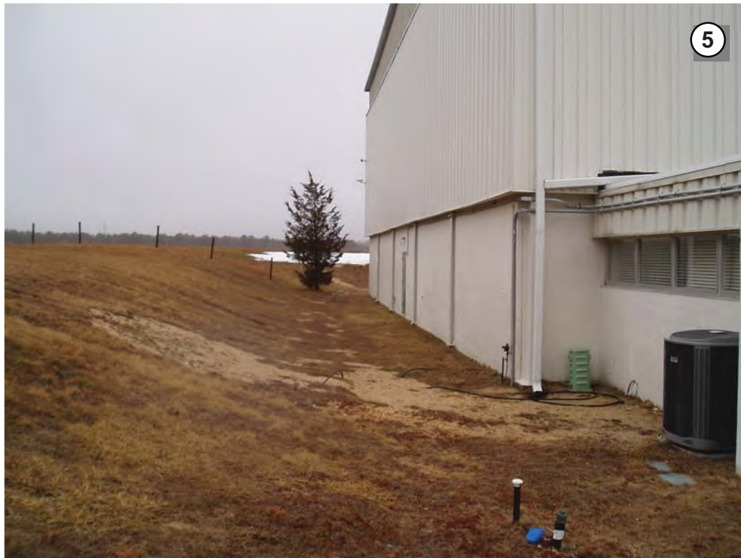
Looking east/northeast at the north façade of Hanger 18. The Preferred Alternative is on the terrace to left. The capped utility lines to the mobile ATCT are in picture foreground (right). (Field Photograph P1010008, February 27, 2013).
