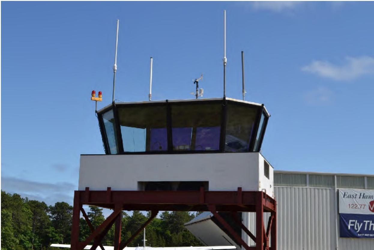
Photograph 2 -1: East Hampton Airport's mobile ATCT, as installed in 2012.
