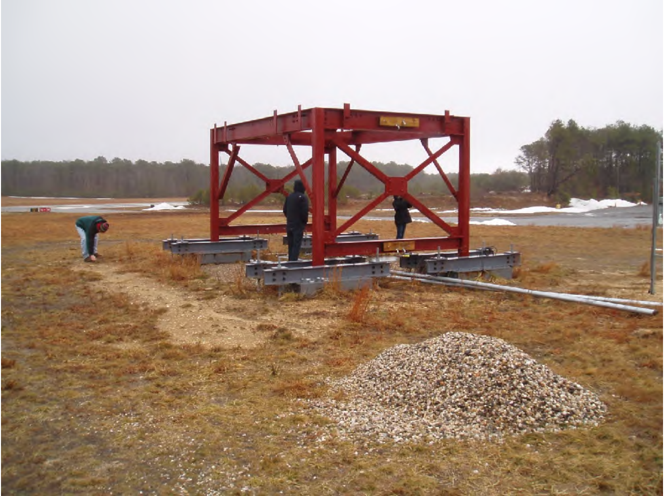
Photograph 2-2: Pedestal structure constructed for mobile ATCT in 2012.
