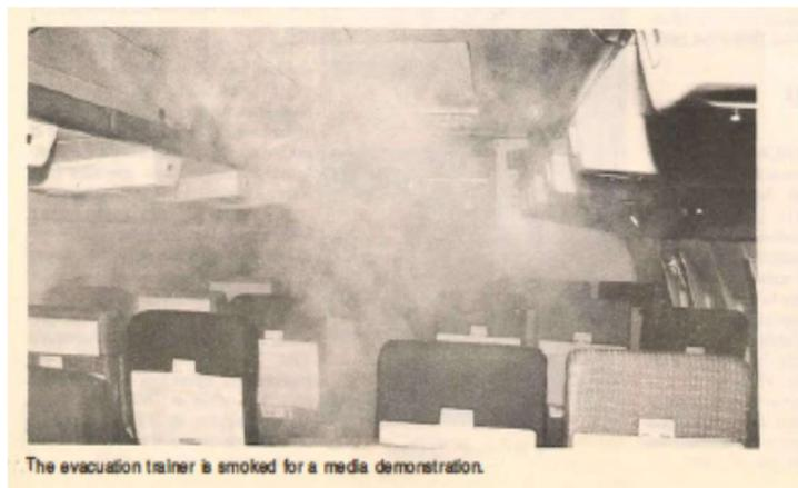
**emergency equipment. This Cabin Trainer was located on an elevated level of the building, which allowed flight attendants to perform actual slide evacuations. The trainer was built upon a massive hydraulic platform, which allowed the trainer to actually move to replicate turbulence. Smoke machines also were also used to fill the cabin with smoke.**
