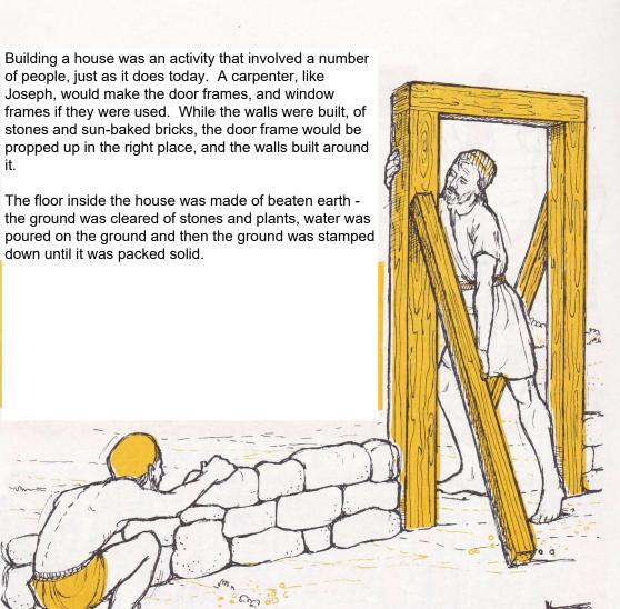
Window frames would be put into the walls as they got high enough, and then the wall finished around them. Where the house owner couldn't afford to have window frames, they would have a lintel - a long piece of stone or wood that would go right across the window opening and into the wall either side, to hold the weight of the wall above the gap.
