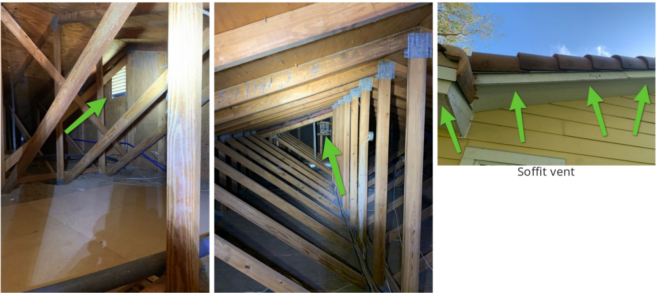
Gable vent. East
