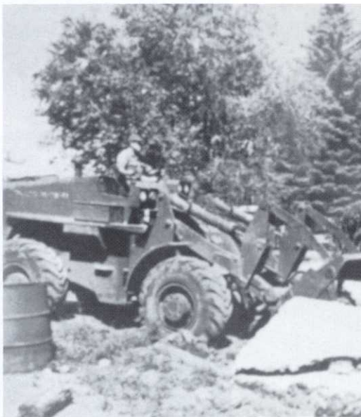
A Fort Carson engineer at work in Center, Colorado.
