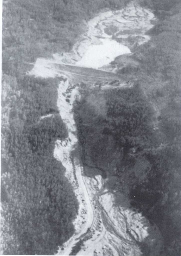
Engineers from Fort Carson complete the Clear Creek Dam project.
