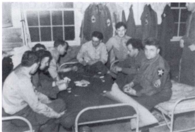
Soldiers filling in time at the transient barracks at Camp Carson, 1948.
