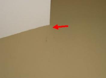
Common small settling cracks in wall and ceiling finish observed. This normal wear for age of home. Recommend repair and paint
