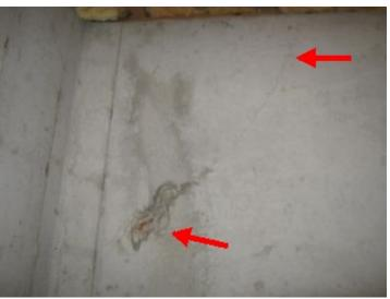
Common cracks. Recommend monitoring over time for increased cracking activity. Recommend sealing of current cracks to minimize intrusion of water/moisture/insects/radon into the building.
