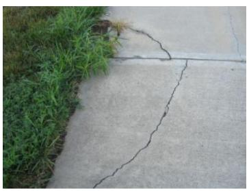
Driveway in good shape for age and wear. Some common cracking/pitting observed. Recommend clean and seal surface to extend life.
