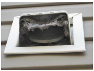
Exterior dryer vent at Northwest corner of house is clogged with lint. Recommend cleaning of unit to minimize fire hazard and improve dryer unit operation.
