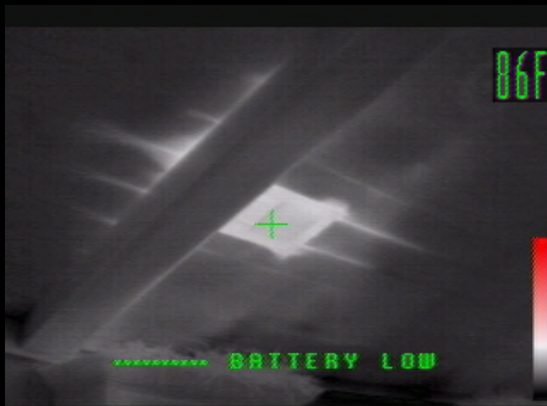
Leaking Ductwork
