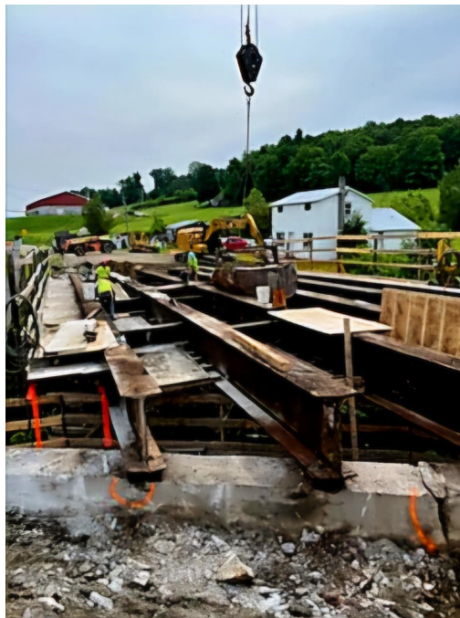
Bridge 6 Deck Removal
