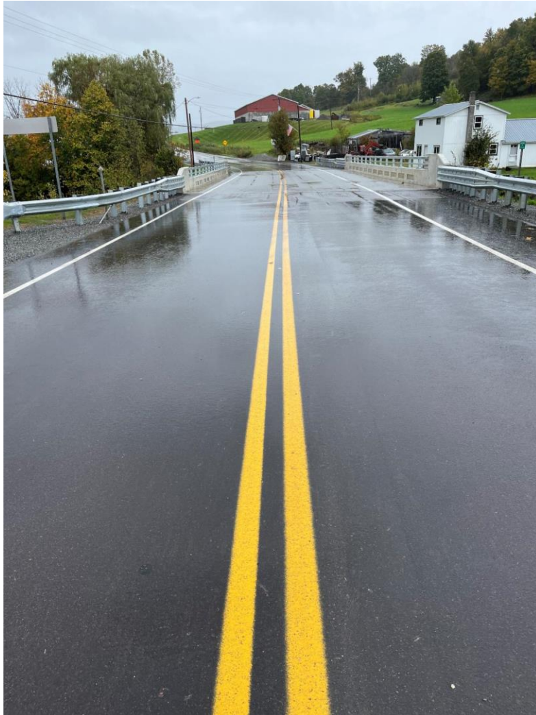
Newly Installed Bridge #6
