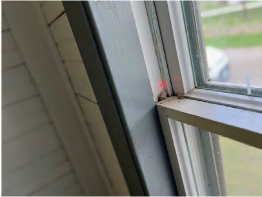
Example of air leak.
