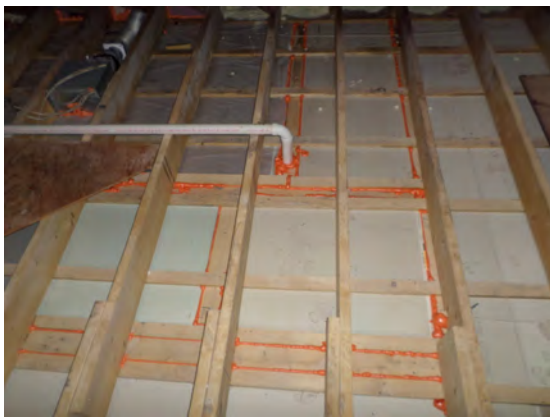
Example of attic air sealing.
