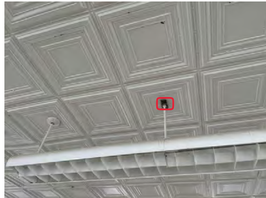
Example of air leak.
