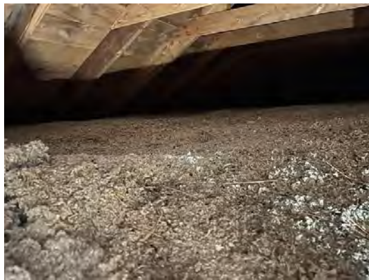
Attic flat insulation, combination of cellulose covering vermiculite.
