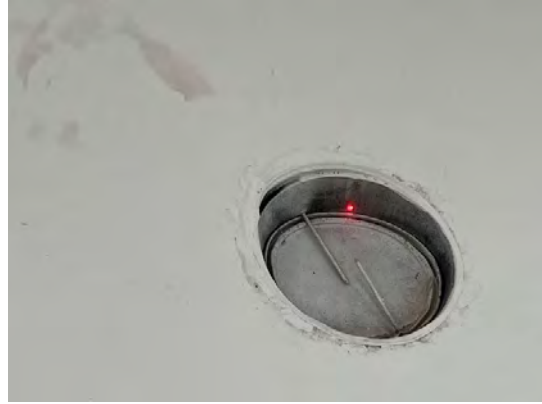
Example of air leak.
