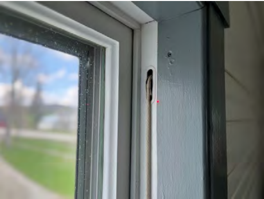
Example of air leak.
