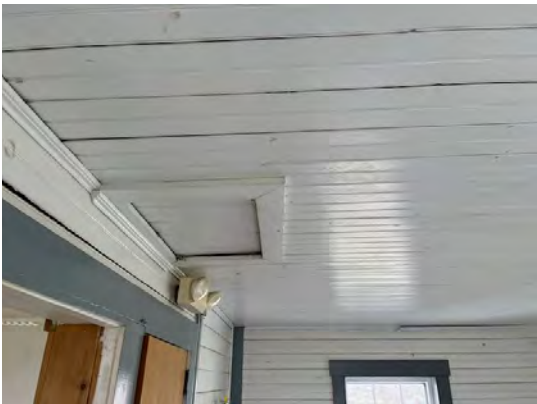
Hatch in stairway section. Tongue and groove boards are leaky.
