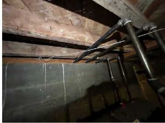
Unfinished basement section. Foundation and rim joist not insulated.
