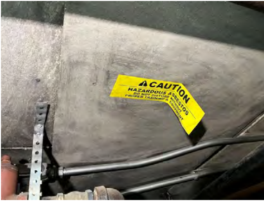
Asbestos hazard sticker in boiler room
