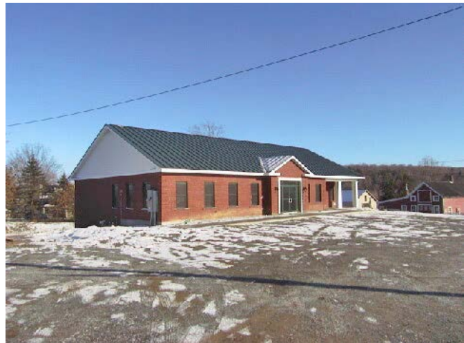
Figure 38 Fairfield Town Office
