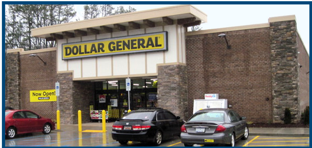
ABOVE: The design of this Dollar General Store, located on Ebenezer Road, reflects modifications suggested at Board of Zoning Appeal hearings.
