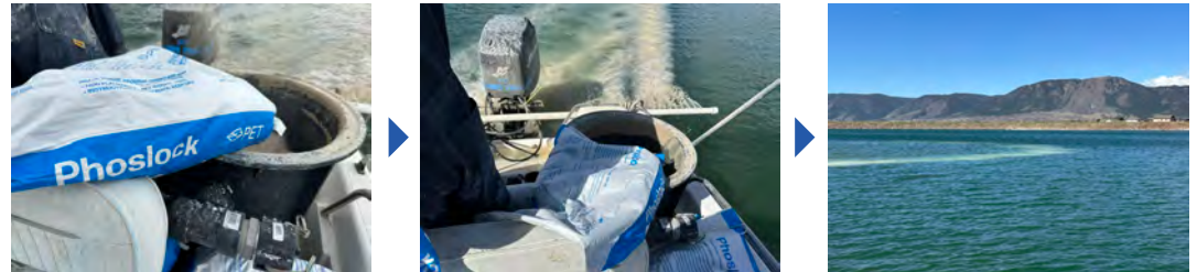
Figure 6. Phoslock® application process, with granules (left) being mixed with lake water (middle) and then applied to the surface of a waterbody (right).
