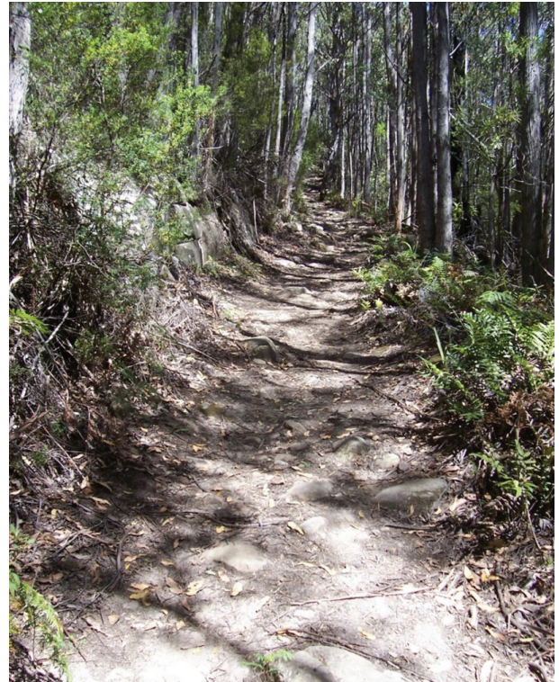
A characteristic section of a simple benched track, on the Fingerpost Track (constructed 1820s). The track has been constructed by cutting into the bedrock on the upslope side. Photo: Anne McConnell
