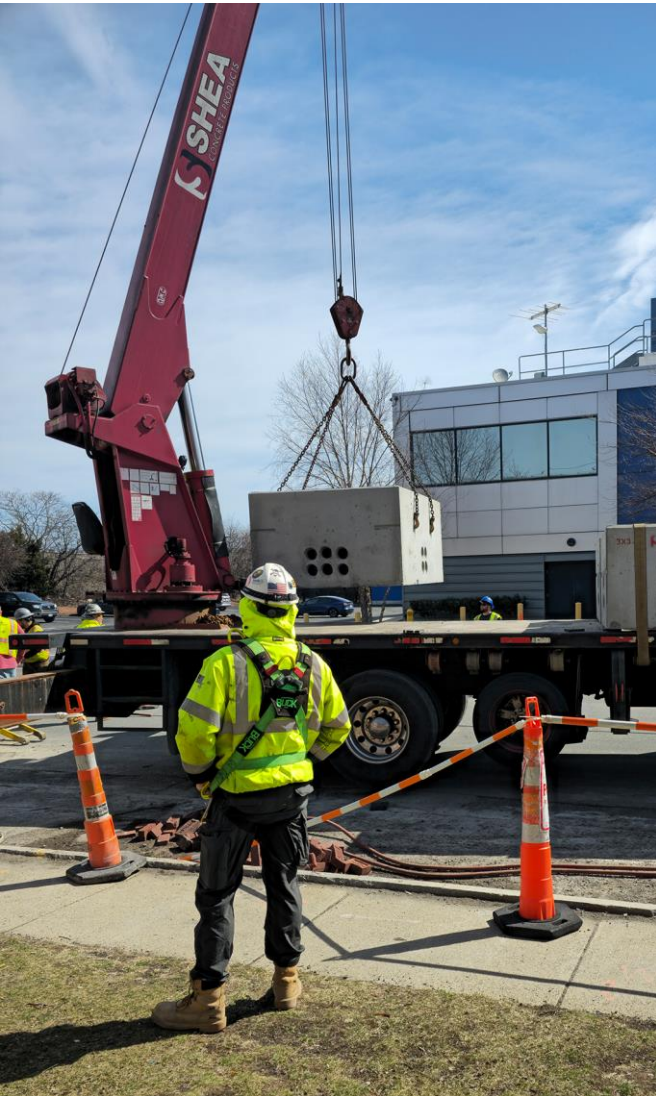
A HEX manhole being installed in 2023. Credit: TWDX Infrastructure
