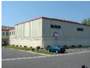
Gymnasium at Faith Academy School of Excellence
