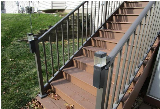
Composite decking with aluminum railings
