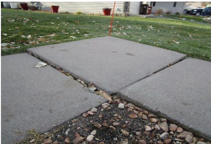
Shifted concrete slabs at a sidewalk
