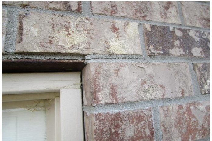
Thin mortar crack
