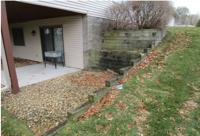
Timber retaining wall with multiple tiers
