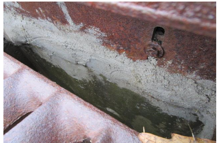
Recent repairs at a catch basin
