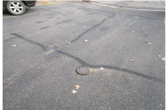
Cracks and previous repairs at driveway pavement
