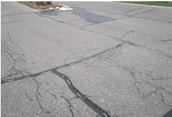
Cracks and previous repairs at street pavement
