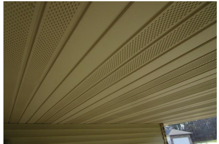
Aluminum soffit with ventilation
