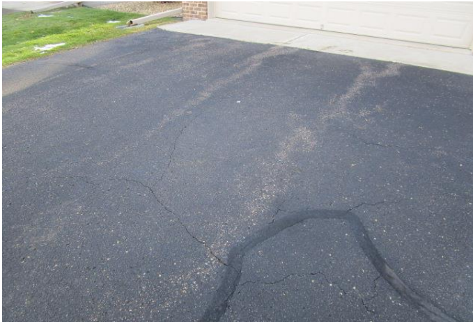
Cracks and previous repairs at driveway pavement
