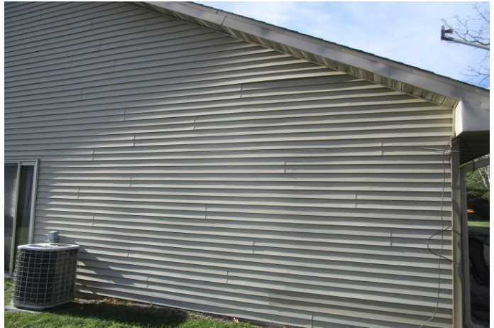
Buckled and warped siding panels
