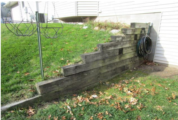
Single timber retaining wall
