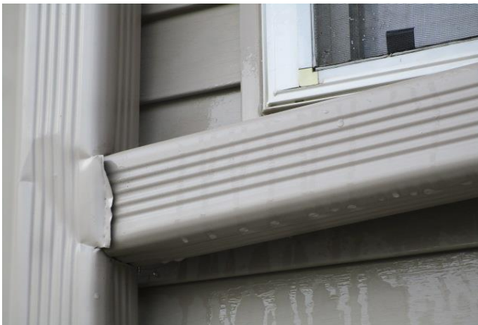
Improper connection resulting in water splashing onto the siding and window - repair through operating budget
