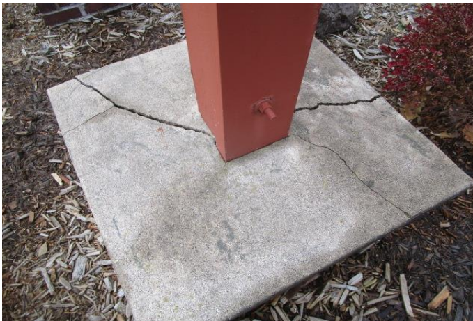
Cracked concrete cap
