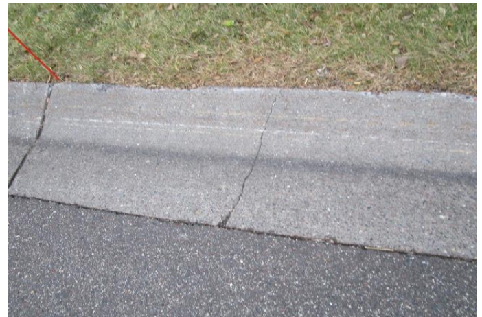
Crack at a curb
