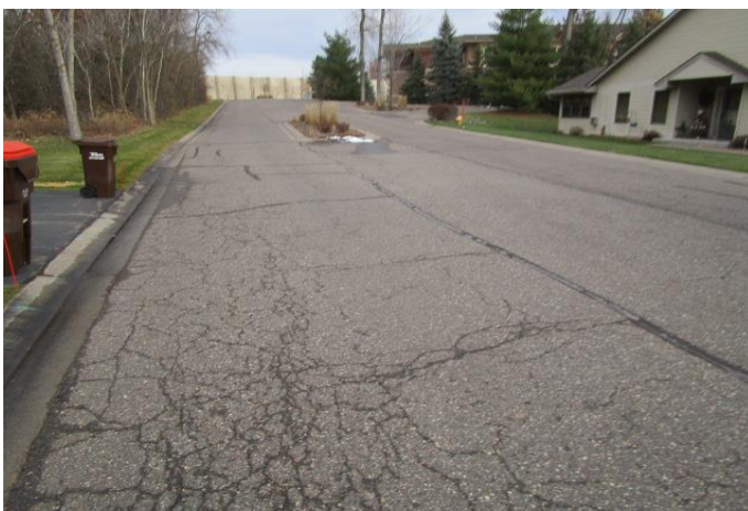
Fatigue cracks and limited crack fill
