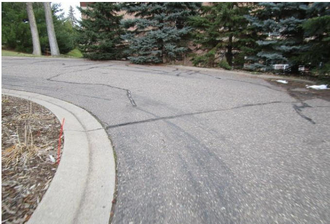
Street overview with cracks
