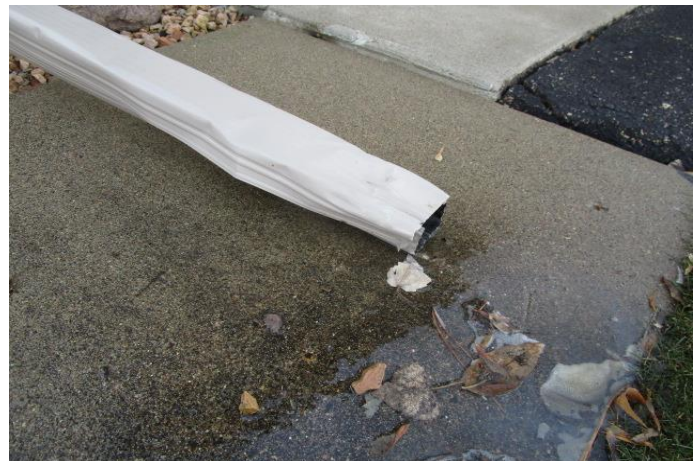
Dented downspout extension - repair as-needed through operating budget
