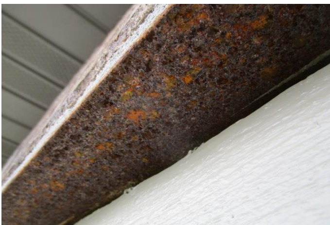
Rust at a steel lintel over a garage door
