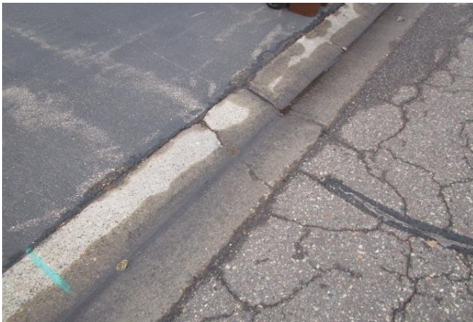
Crack at a curb
