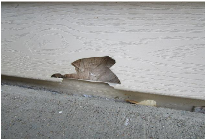
Damaged siding panel showing exposed wood sheathing
