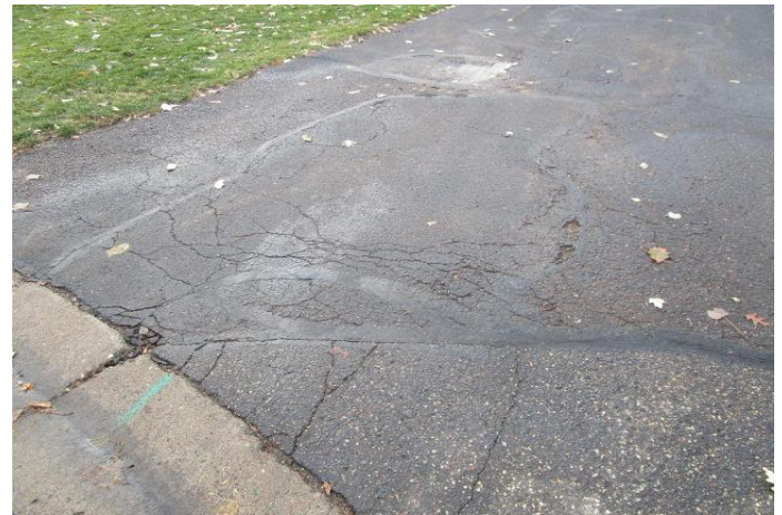
Fatigue cracks at a driveway
