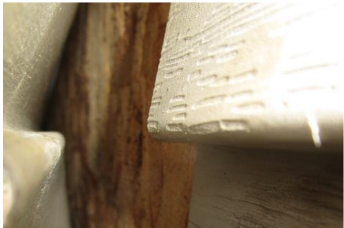
Spot checks behind siding revealed a lack of waterproof barrier
