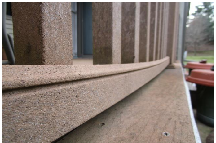
Detail view of composite railing with sag
