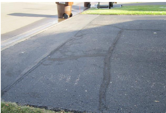
Crack fill, cracks and a previous patch
