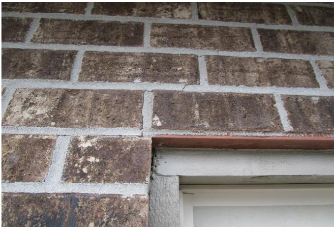
Thin mortar crack
