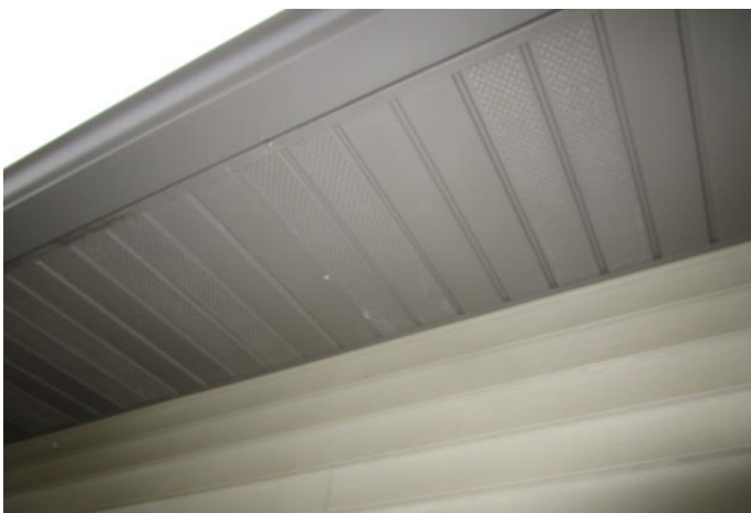
Vented soffit
