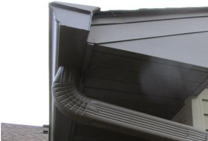
Gutter and downspout connection
