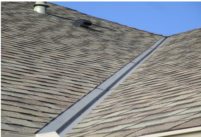
2012 roof with metal valley flashing
