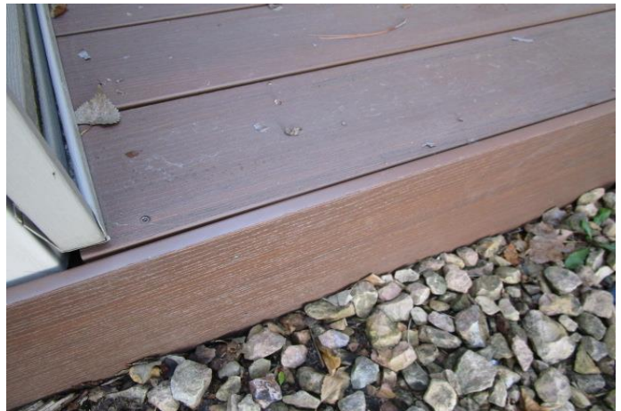
Decking and fascia are composite
