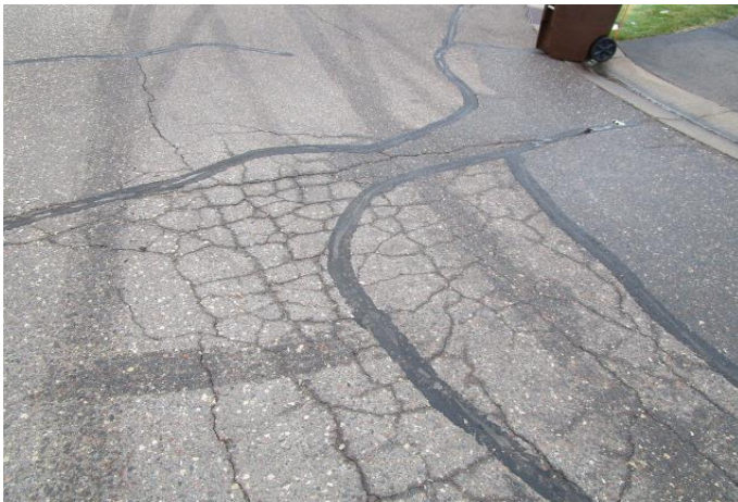
Fatigue cracks and previous crack fill
