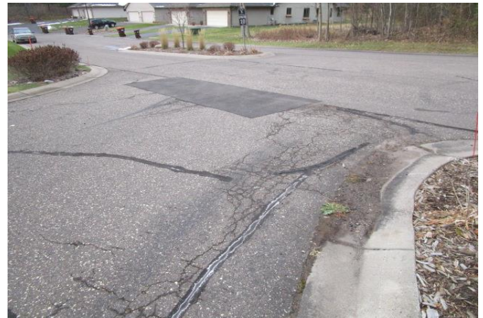
Fatigue cracks and a patch
