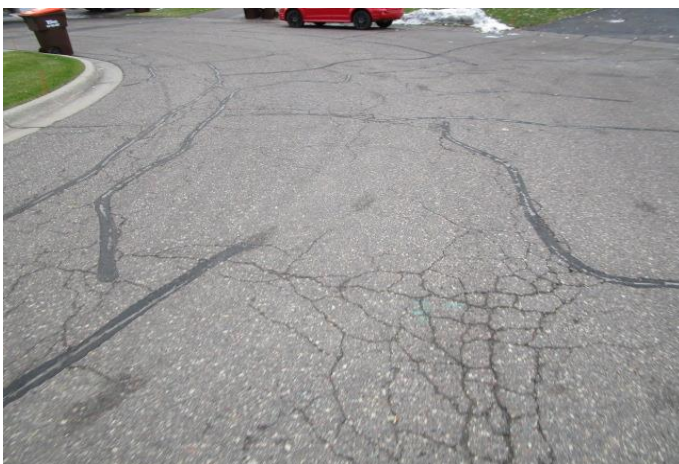
Fatigue cracks and limited crack fill
