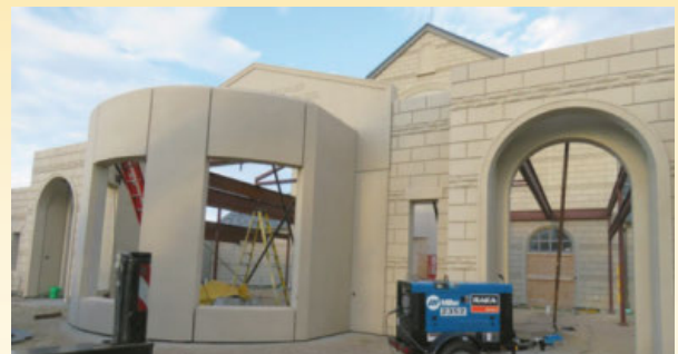
Progress as of August 28th
