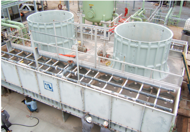
1. Preparing existing cooler for expansion
