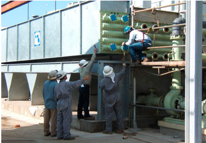
3. Additional tube bundle installed
