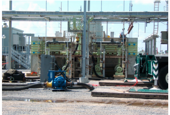
4. Expansion of existing cooler complete
