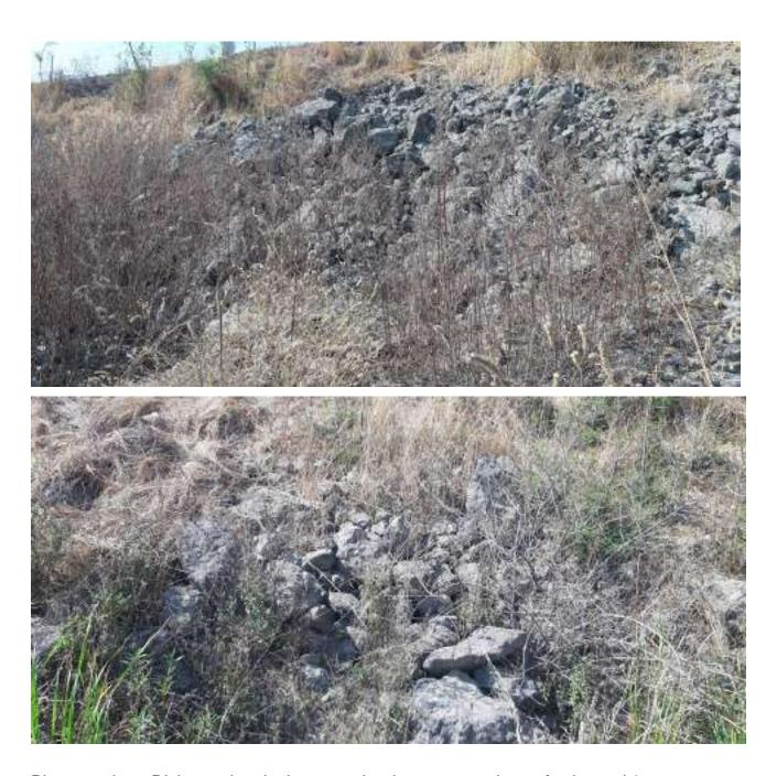
Photograph 5 : Dislocated rock pieces on the downstream slope of ash pond 2
