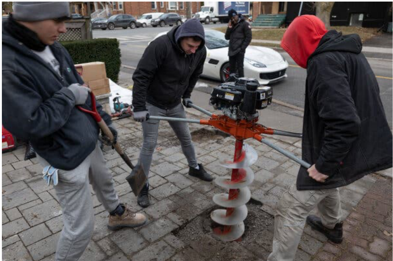
Workers from Bollard Boys GTA installing a bollard in a driveway in Toronto. Credit... Ian Willms for The New York Times
