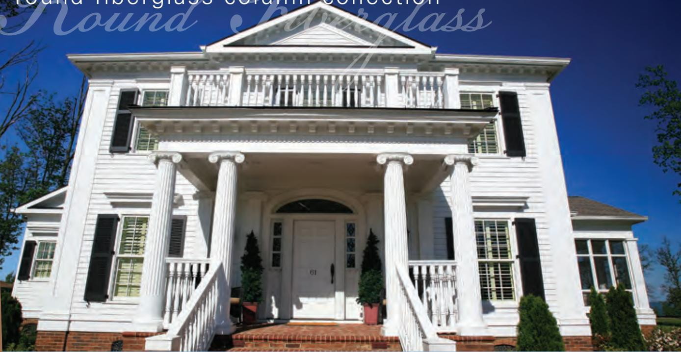
Master craftsmen closely control the preciseness of entasis, projections and profiles for accurate detail. Round and square fiberglass columns are available in plain and fluted shafts. Decorative capitals are manufactured from a composite mold of marble and polyester resin. Resin-infusion columns are lightweight and durable and make an excellent choice for projects featuring large exterior columns. ABling also specializes in historical replications.
