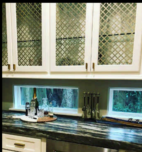
Designer Perforated Metal, CLASSIC 2058, Carbon Steel, Cold Rolled, 20 Gauge (.0359" Thick), 58% Open Area used as cabinet inserts.
