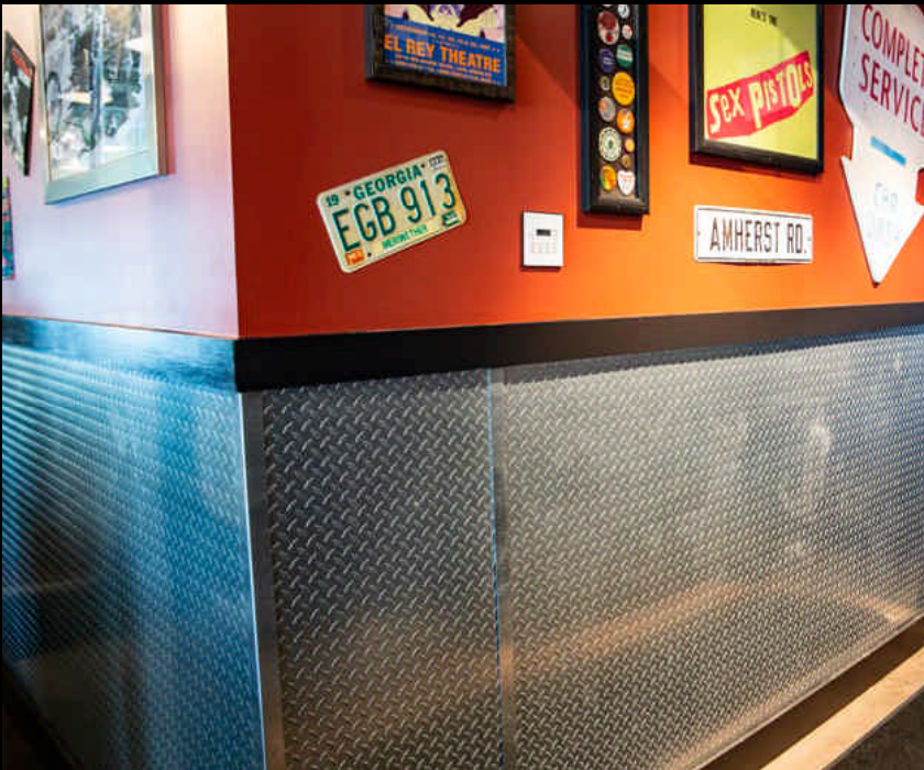
Textured Metal, Designer Textured, TREADTEX® 1400, Aluminum, Alloy 3003-H14, 2-B Finish, .0630" Thick (14 Gauge), is used as wall cladding to create an industrial feel at this regional burger joint.
