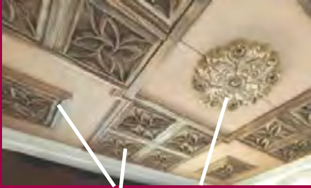
Ceiling Tiles and Medallion
