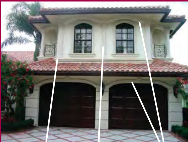
Molding and Columns w/Corinthian Caps Arches w/Keys around garage doors and windows
