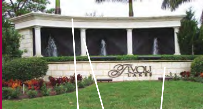
Entry Wall with Molding, Columns and Wall Treatment
