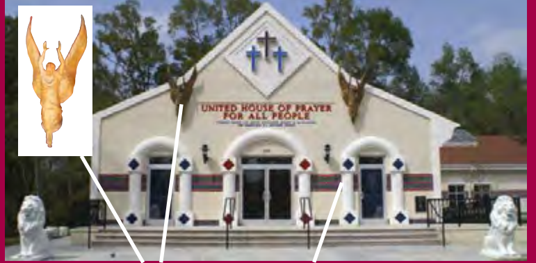
Molded Angels and Arch Entryways with Columns
