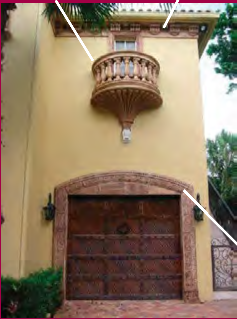
Window Balcony w/Balusters & Brackets under eave
