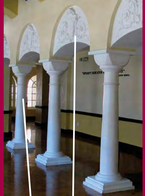
Columns and Arches with Appliques
